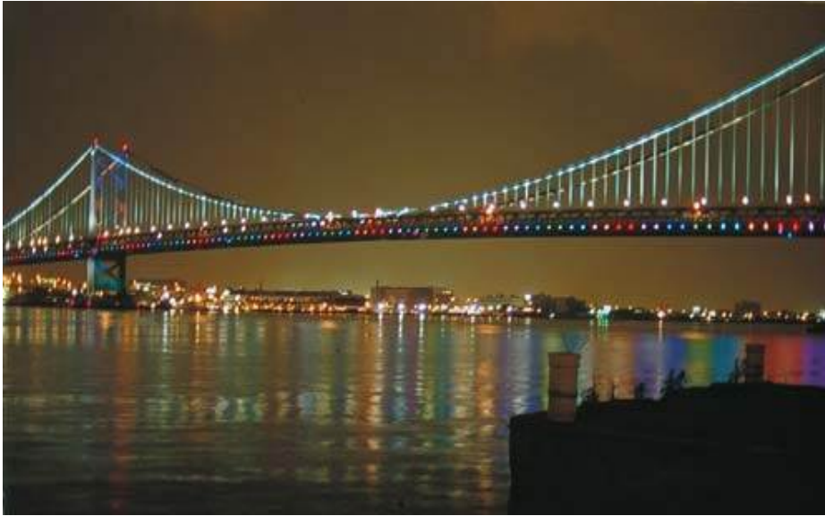
LED Installation Benjamin Franklin Bridge, PA, USA (Color Kinetics Inc.)
